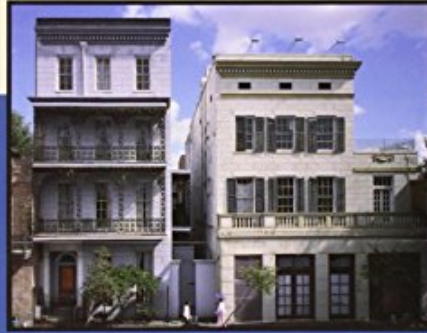
The same two buildings, 1993
